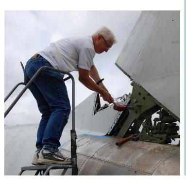
Painting of 081 has begun. The vertical tail has been painted with the required 3 color camouflage (dark green, medium green and tan) and the bottom of the fuselage has been painted light gray.
