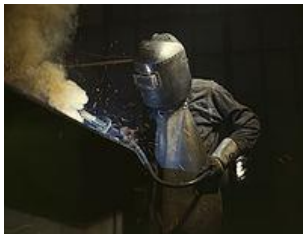
Welder making boilers for a ship, Combustion Engineering Co., Chattanooga, Tennessee. June 1942.
