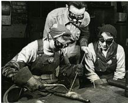
Brazing at the Gary Tubular Steel Plant
