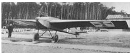
In secret, the Junkers J 1 undergoes engine running in December 1915 before its pioneering flight tests, as the world's first practical all-metal aircraft.
