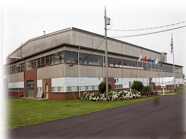
Before the brickwork
