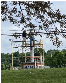
Scaffolding erected in preparation for Jean Ann II's return
